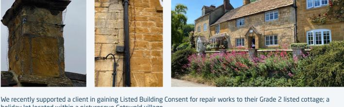
The proposals included the replacement of a crumbling chimney, alterations to the roof (including retiling, provision of additional insultation and ventilation, along with new rooflights). The front elevation of the property also needed
